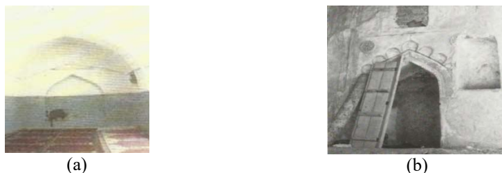
Figure 40: Wall gaps is called “Al-Faregha.” (a) The gap in the walls of Al-Jumah Mosque (Source: Al-Haddad, 2004); and (b) The gap in the wall of Al-Qara Mosque in Al-Ahssa (Source: King, 1986).
